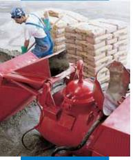
Mixing Topcem with an automatic pumping unit
