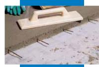
Detail of a Topcem screed with reinforcement rods
