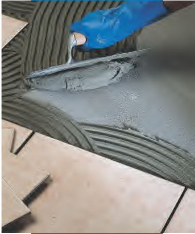
Installation of single-fired tile on floor
