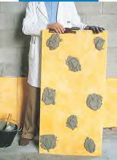
Spot-bonding insulating panels on untreated wall
